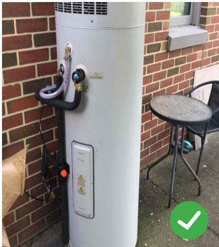
Figure 6: The drain is run from the container away from where the TPR will be operated.
