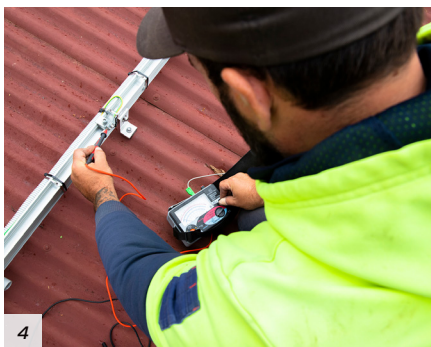
5. Ensure all SWMS are planned and prepared as per WorkSafe Victoria requirements.
