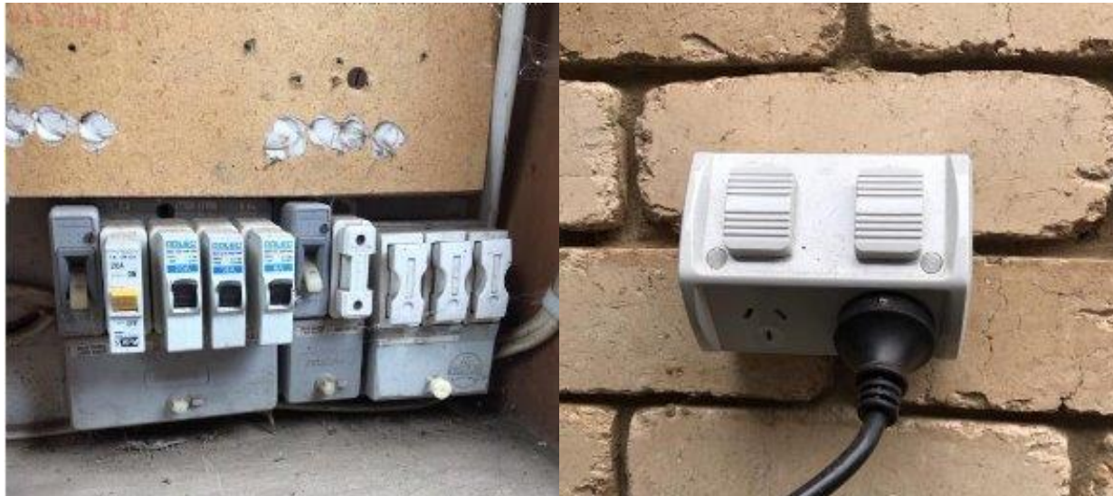
Socket outlet installed for purpose of heat pump supply not protected by an RCD.
