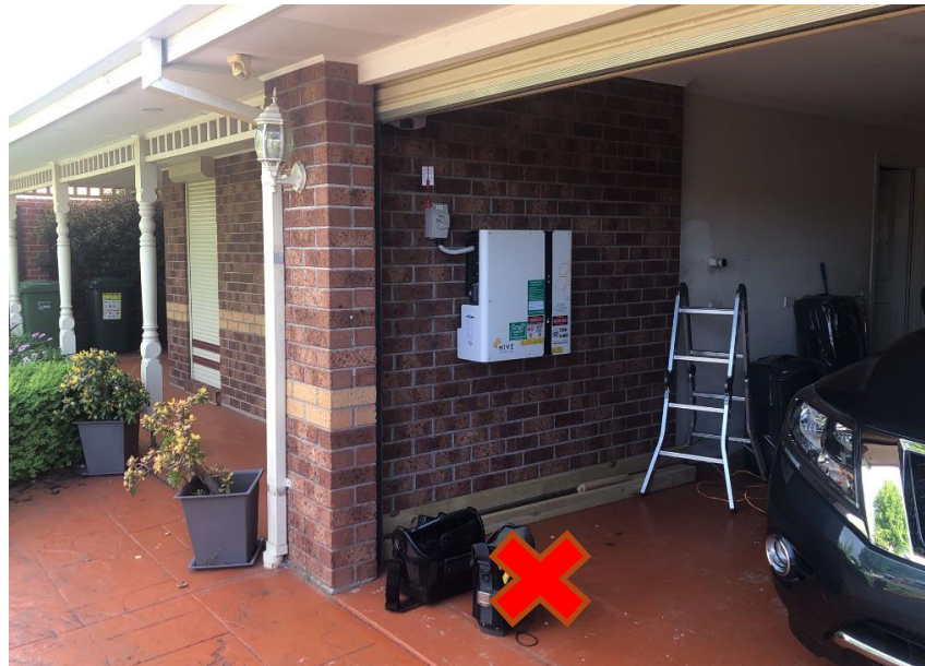
Fig. 1 Standard Double Garage 6m x 6m Standard Single Garage 4m x 6m Area requiring Additional Mechanical Protection (such as a Bollard) Area deemed protected by the garage pillar or wall, not requiring additional protection. As a guide the protected area is calculated at ratio 1 : 2.5 i.e: 500mm garage pillar, would allow an area of 1250mm protection along the wall. Each installation must be assessed for potential hazards and any reduction methods implemented.
